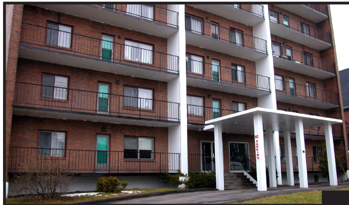
CARLETON TOWERS 15 Mecklenburg Street, Saint John, NB
