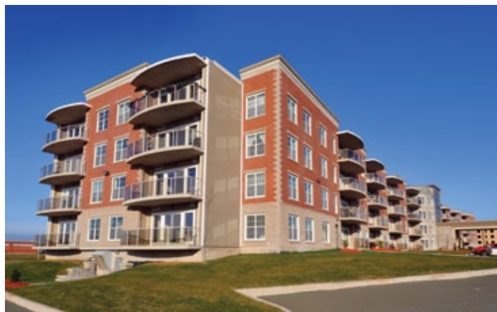
(1) 180 Mill Street is a 127-unit property. Killam owns a 25% interest, representing 32 units
