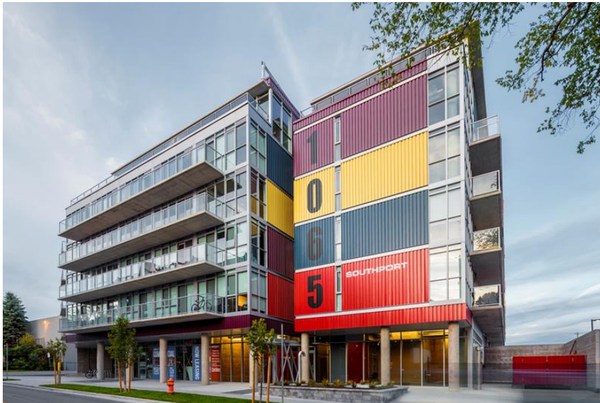
Southport, Halifax – Completed 2016
