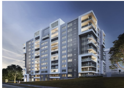
The Kay | 128 units Mississauga
