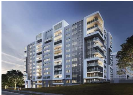
The Kay | 128 units Mississauga
