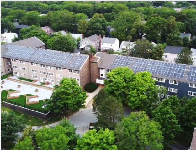
Quinpool Court | 2155 & 2225 Monastery Lane, Halifax, NS 94 kW array | 113,000 kWh annual production | 7.7% return on investment (ROI)
