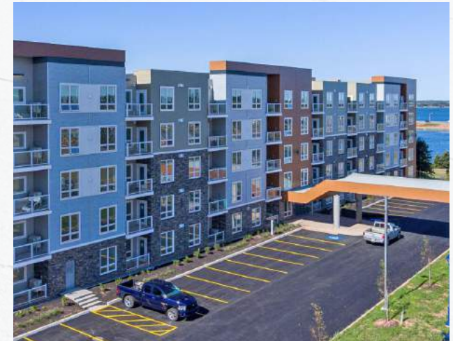
Shorefront | 31 Michael Thomas Way, Stratford, PE 100 kW array | 111,000 kWh annual production | 6.4% ROI
